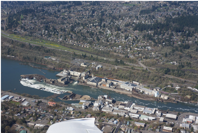
Photo: Aerial view of Willamette Falls Locks
